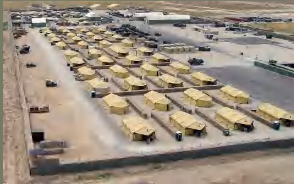
All surrounding protection of the Military Base
