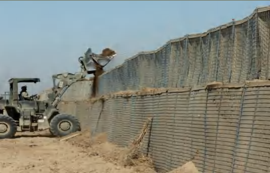
Construction of the Barrier
